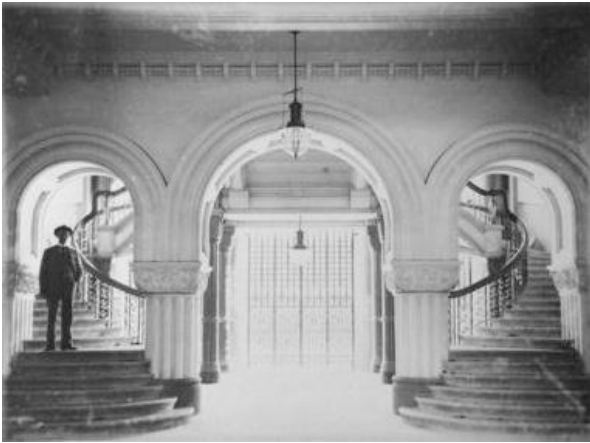
Figure 27 – Looking out to the street from the central dome area, 1898
