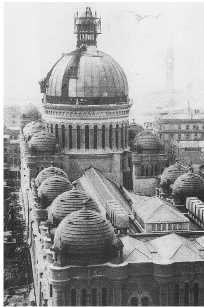
Figure 25 – The central dome nearing completion, c. 1898
