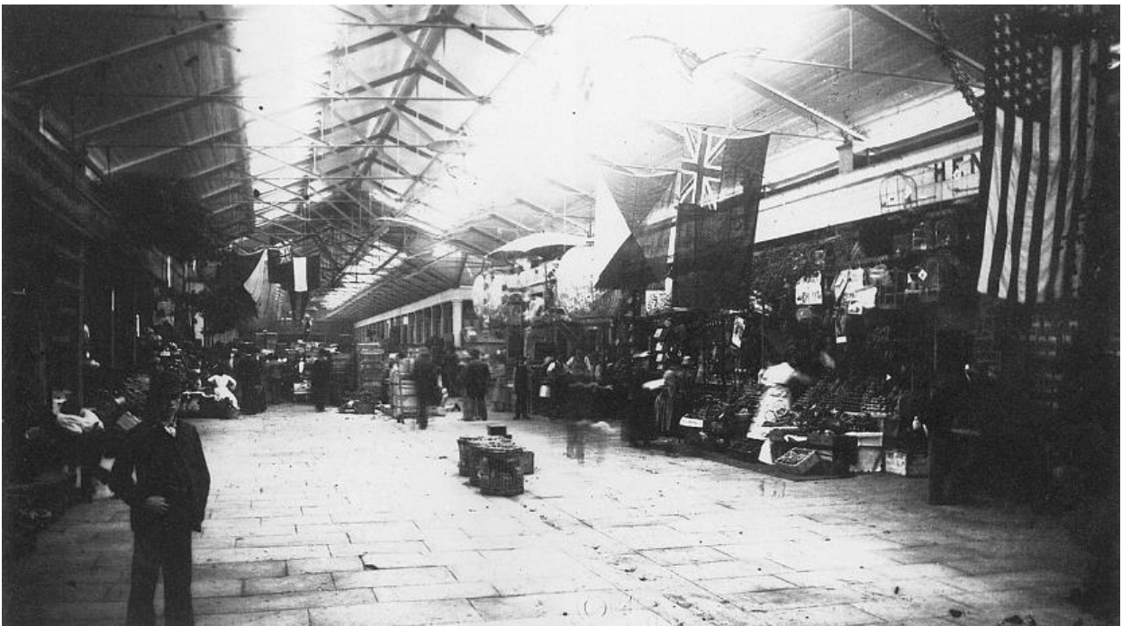
Figure 12 – Interior view of the George Street Market, undated
