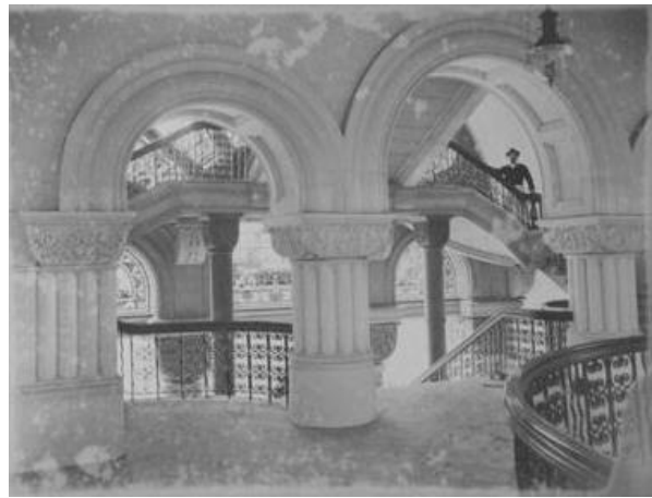
Figure 28 – Looking into the stairway leading off the central dome area, 1898
