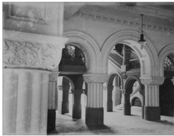
Figure 30 – Looking into the stairway leading off the central dome area, 1898
