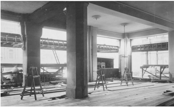
Figure 47 –The ground floor tessellated tiles were concealed under concrete and timber, 1918
