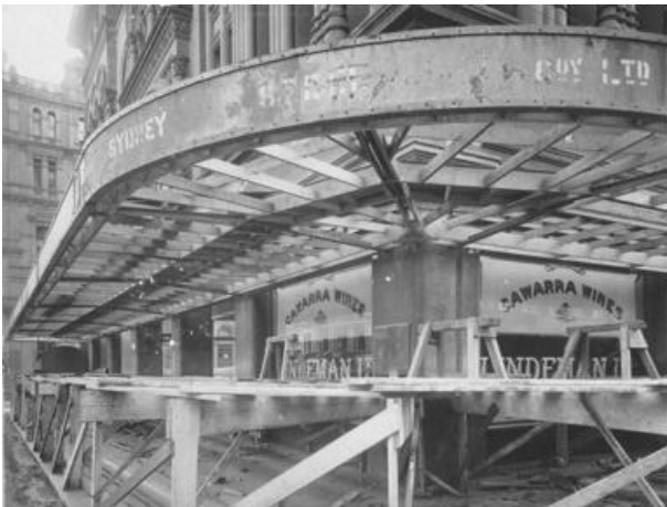
Figure 41 – Images of the 1918 alterations. Construction of the steel cantilevered awning, 1918
