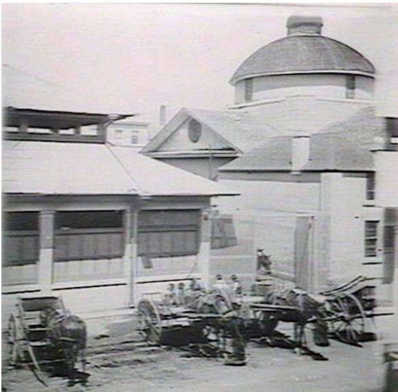
Figure 10 – George Street Markets with Greenway's Police Court building to the right, pre-1891
