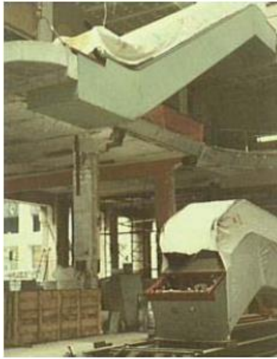
Figure 77 – Escalators were installed in the north and south voids in 1985
