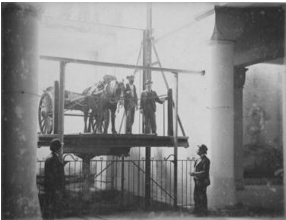
Figure 31 – One of the York Street lifts which serviced the basement livestock, fruit and vegetable market, 1898
