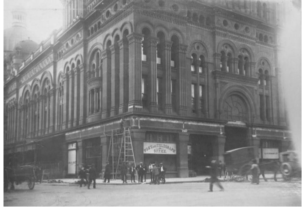
Figure 40 – Images of the 1918 alterations. Removal of the posted awning, 1918
