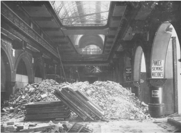
Figure 43 –Internal demolition, 1918 Source: City of Sydney Archives, NSCA CRS 51/2300
