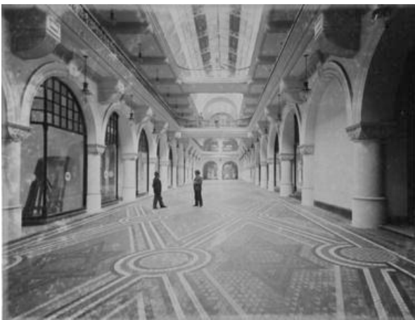
Figure 29 – Looking through the ground floor of the galley with decorative tessellated tile floor, 1898
